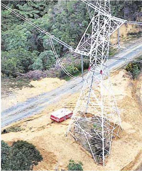
Figure 4 HOLDING ON: Red clamps halfway up the power pylon, with four steel guy-ropes that are embedded in concrete in the ground, help maintain the South Island's electricity flow. NZ Herald graphic 30 August 2008
